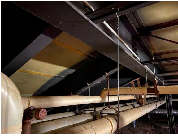
Photo #9: Roof structural steel from catwalk
