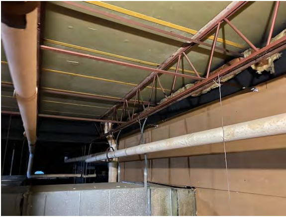
Photo #10: Roof bar joists above mech room
