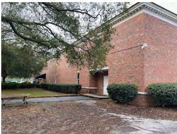
Photo #4: Northwest Corner
