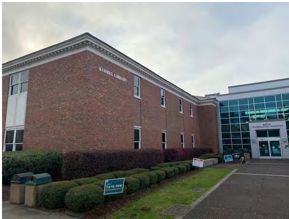
Photo #2: Southwest Corner
