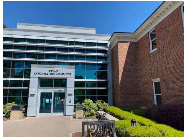
Photo #6: Existing to Newer Bldg Interface
