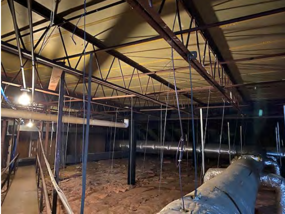
Photo #11: Roof bars and mechanical hangers
