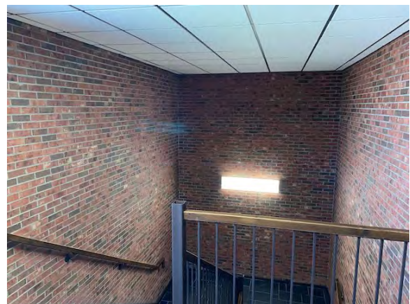
Photo #8 - Northwest stairwell
