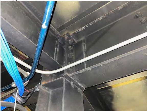
Photo #12: Structural column and beams at Flat roof corner
